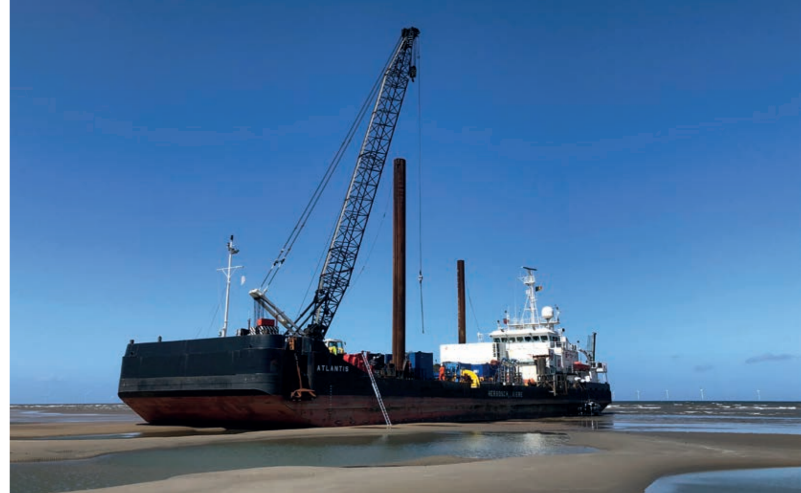
Repair of subsea cable using the ATLANTIS, Liverpool.
