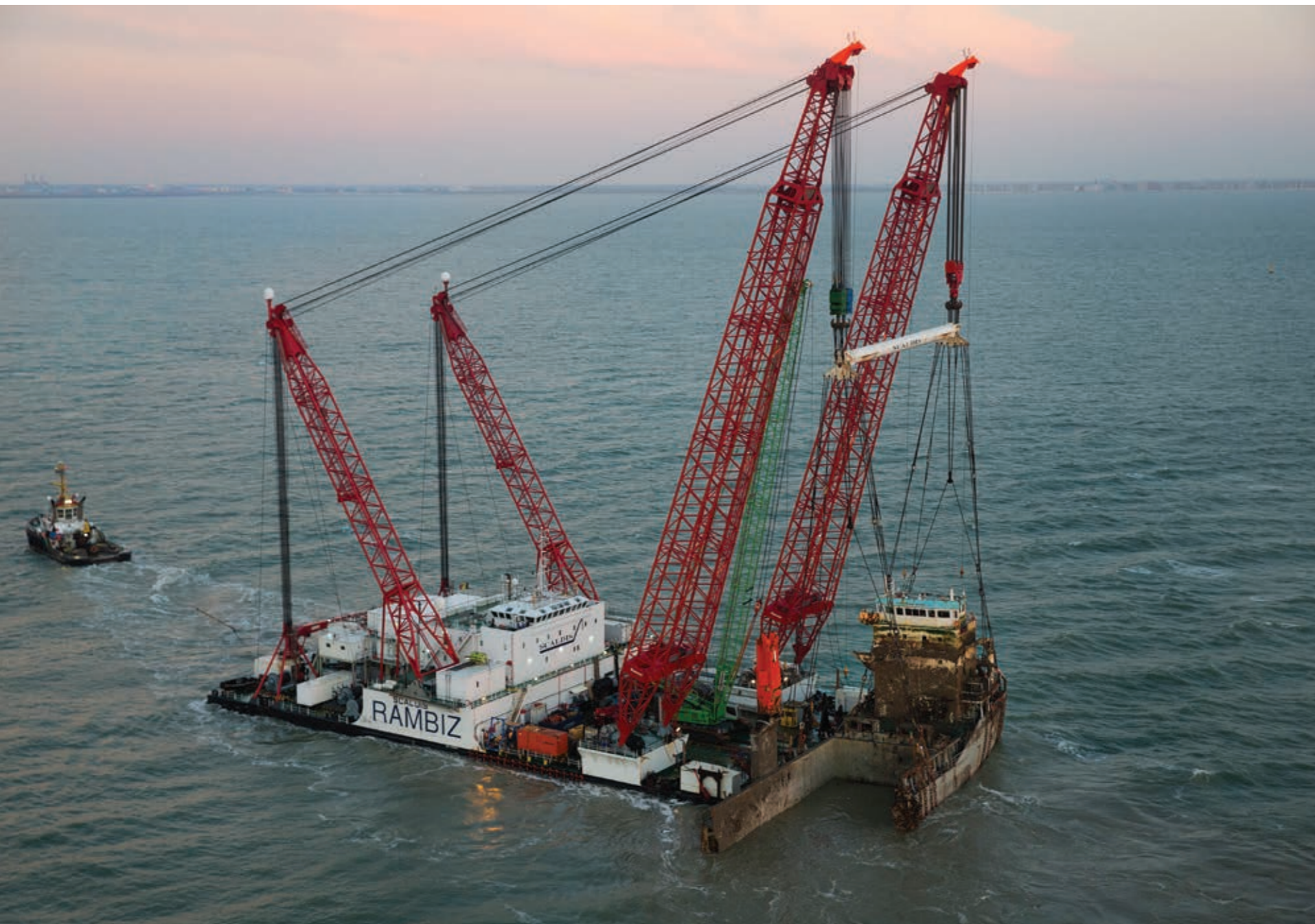
Salvage of the cargo of the Flinterstar with the RAMBIZ, Belgium.
