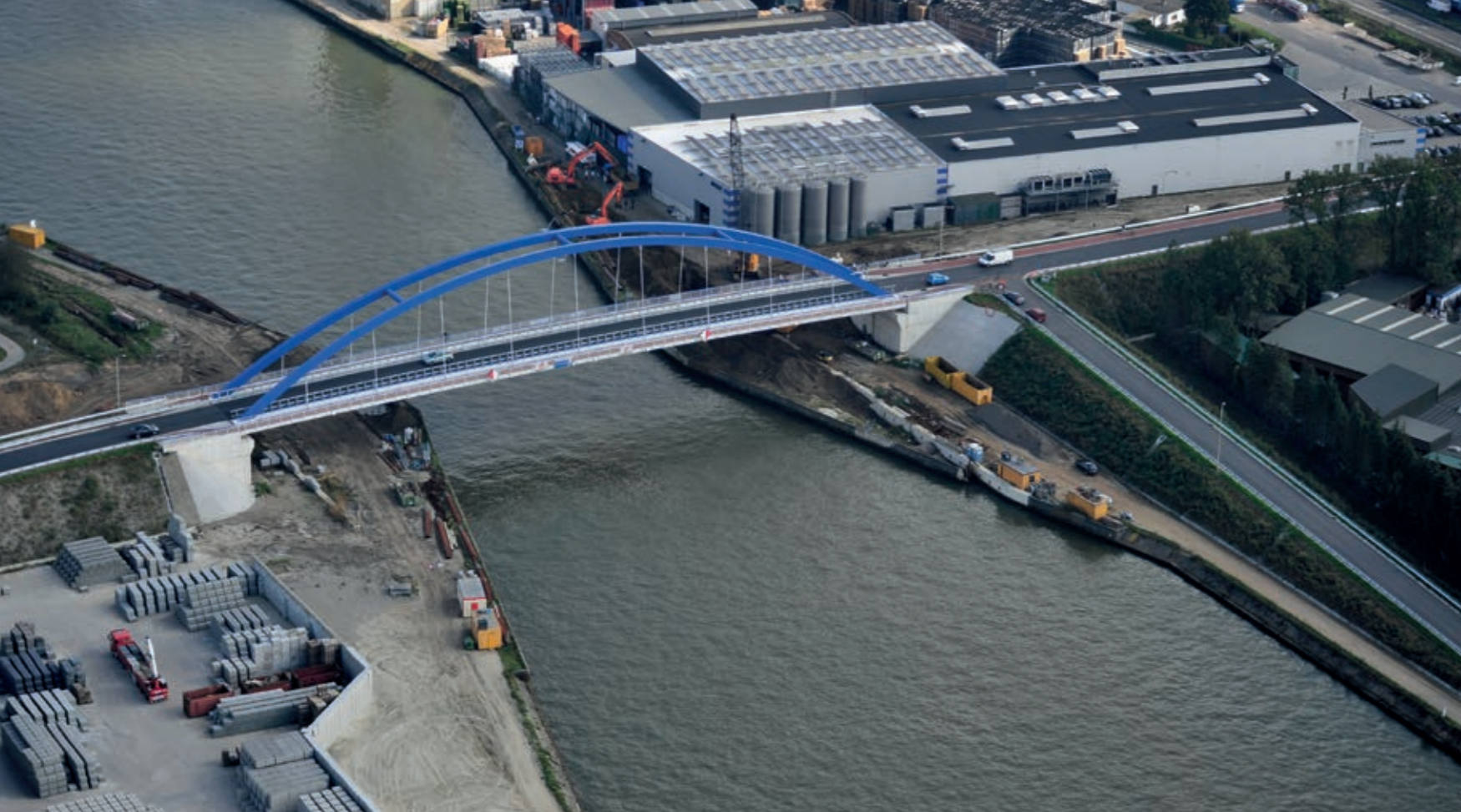
Demolition and construction of a bridge over the Albert Canal, Belgium.
