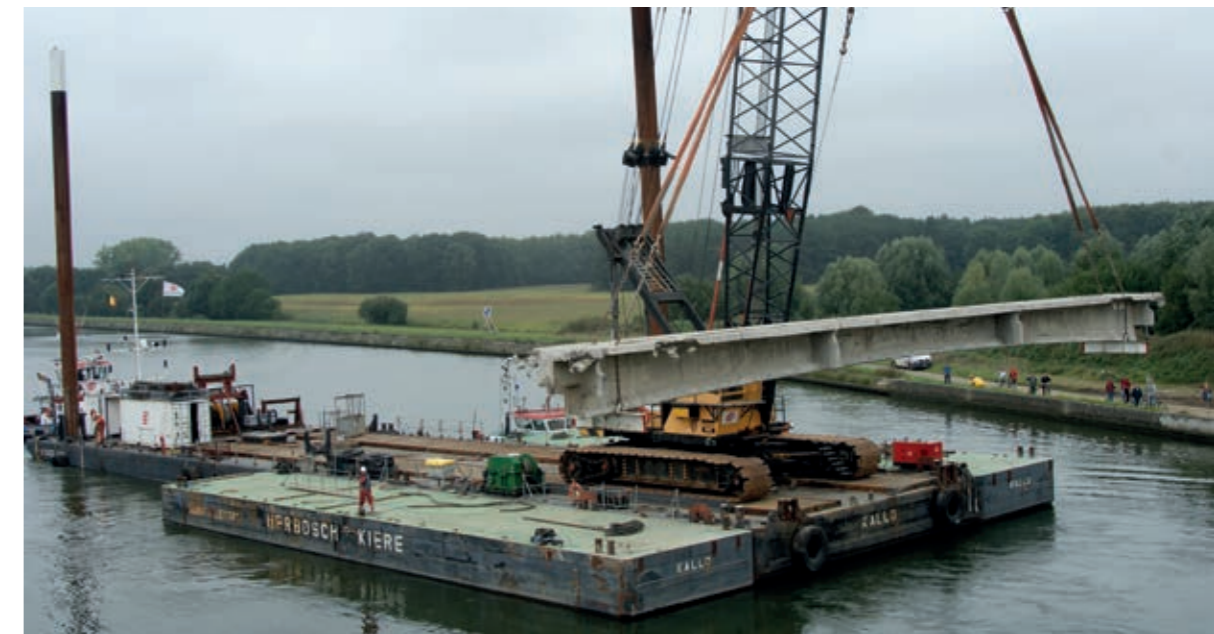
Demolition and reconstruction of a bridge in Viersel, Belgium.
