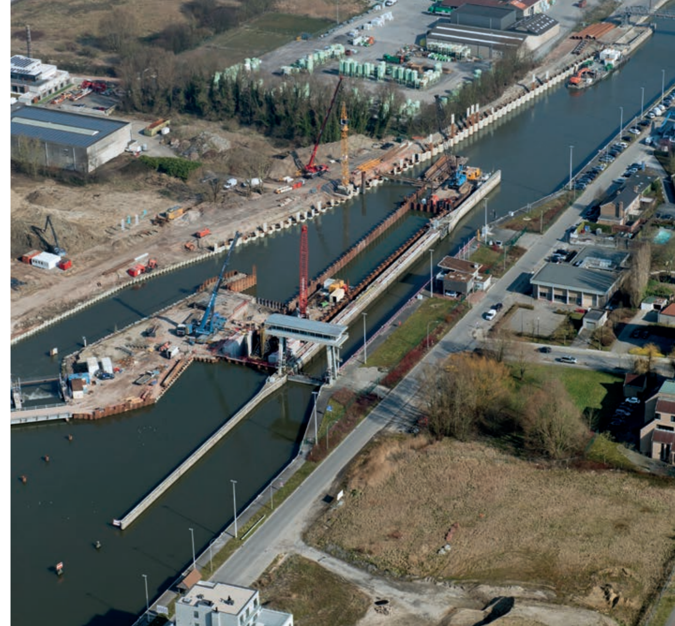
Design and construction of a new lock weir in Harelbeke, Belgium.
