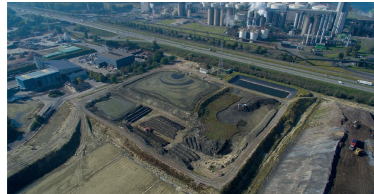
Waste treatment and coverage in Ghent, Belgium.
