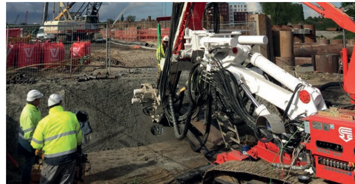
Installation of micropiles as foundations for the lock in Harelbeke.
