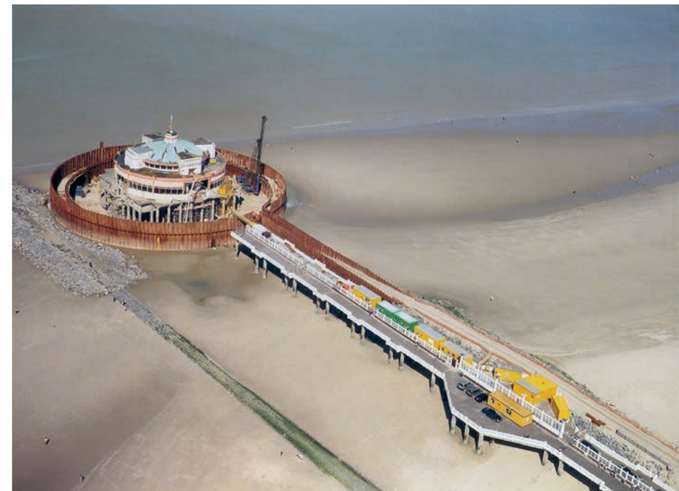
Piling works for the renovation of Blankenberge Pier, Belgium.
