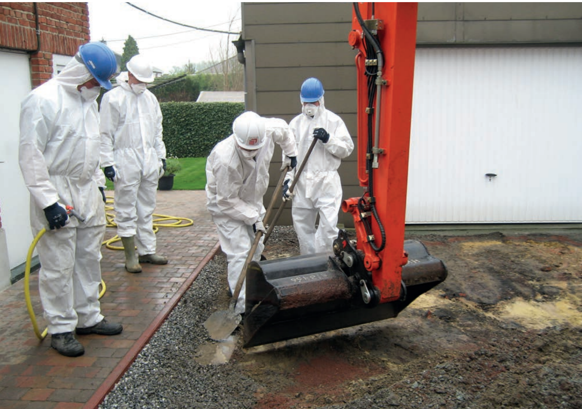
Asbestos removal, Belgium.
