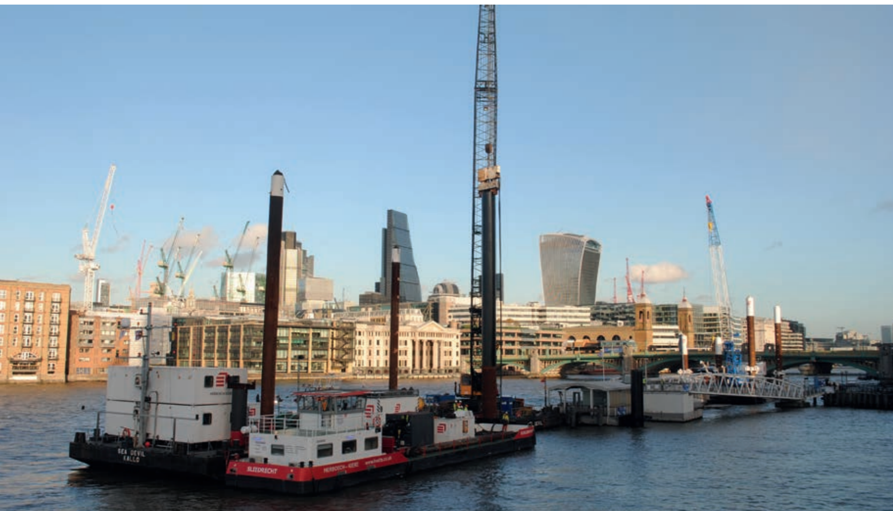
Extension of Bankside Pontoon in London to give more boats access to the pier.
