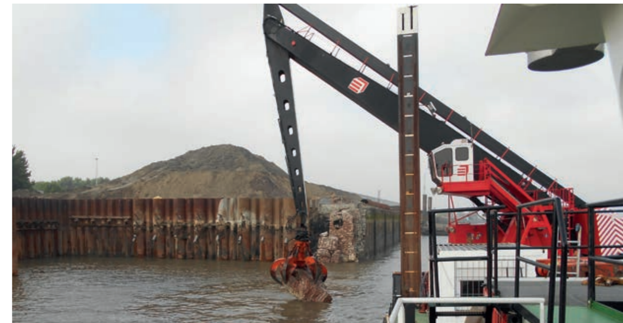
Demolition of a 700m quay wall in the Scheldt, Belgium.
