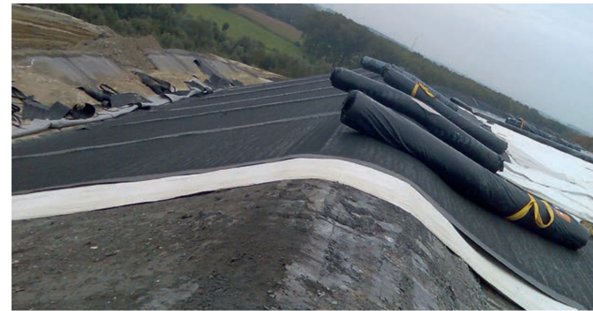
Waste treatment and coverage in Ghent, Belgium.
