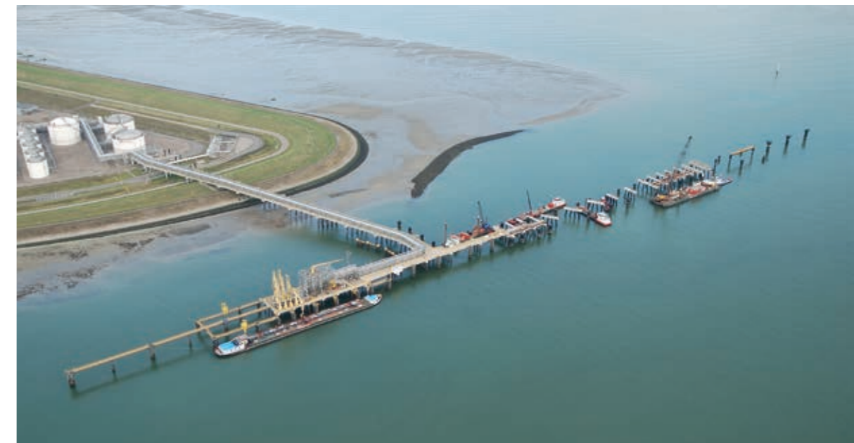
Construction of a sea jetty in Terneuzen, Netherlands using the Atlantis.
